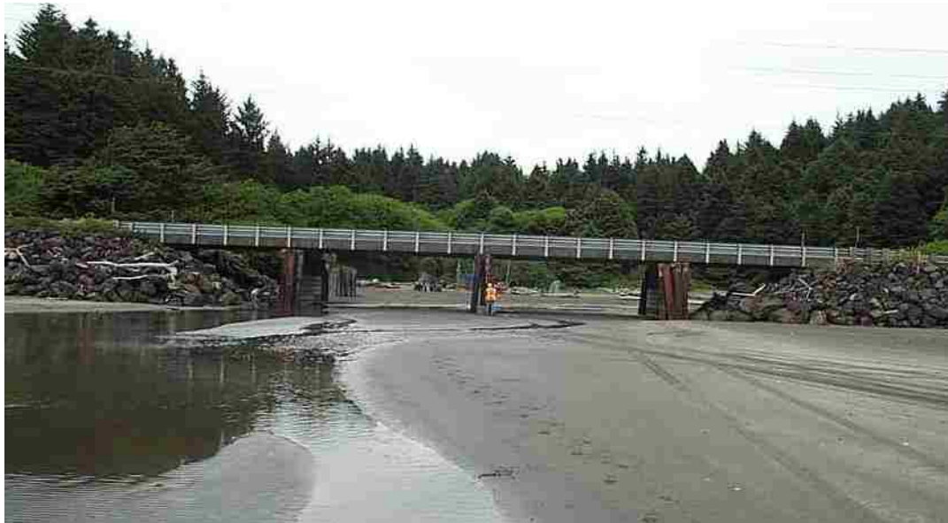
Figure 6-2: Wreck Creek Bridge (WSDOT, 2003)
